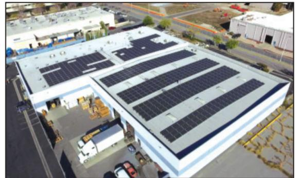
Mitsubishi Electric solar modules cover Mortech Manufacturing's facility. The 183.4 kW installation is in Azusa, Calif.
