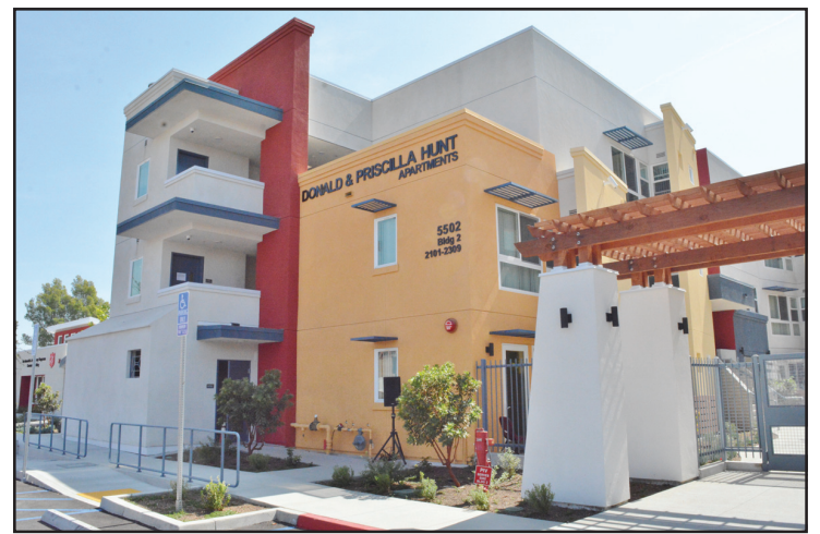
The Salvation Army Donald & Priscilla Hunt Apartments at Bell Oasis. Funds. All units, except the manager's unit, are subsidized by Project-Based Vouchers from the CDC/HACoLA.
